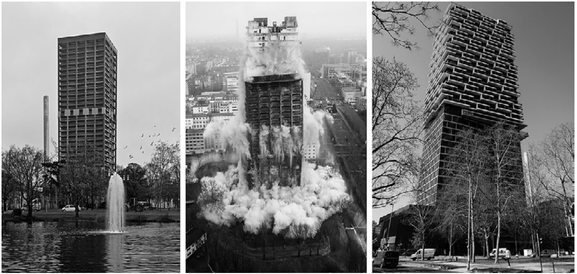
Figure 2. Left: AfE-Tower in Frankfurt/Main before its demolition in 2014 (Image credit: Karsten Ratzke, image placed in public domain). Centre: Demolition of AfE-Tower in February 2014 (Image credit: Sven-Sebastian Sajak, licensed under CC BY-SA 3.0). Right: One Forty West building in March of 2021 (Image credit: User 'Silesia711' through Wikimedia Commons, licensed under CC BY-SA 4.0)
