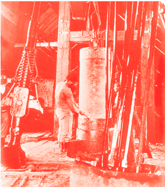
Figure 7. Drilling, Inserting Iron Pipes Into a Well, n.d., photograph, accessed November 29, 2025, pinterest, https://www.pinterest.com/pin/390757705172188838/
